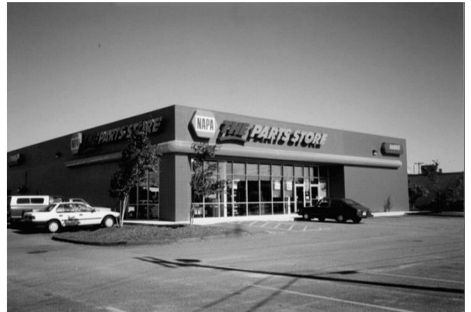
This building pays little attention to the site where it is located, nor gives much attention to detailing and the roofline. Flat roofs such as this are discouraged.
