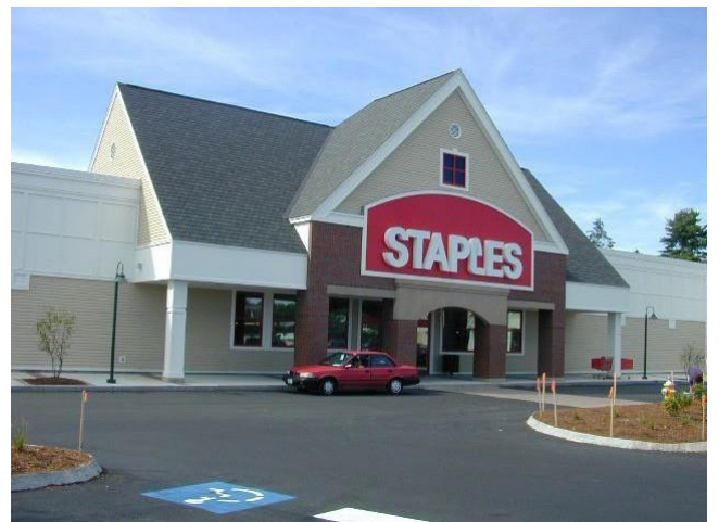
A similar building with a facade composed of New England forms and materials. The overhang provides protection for pedestrians and emphasizes the entranceway. The sign is over scaled (i.e., too large) for the facade.
