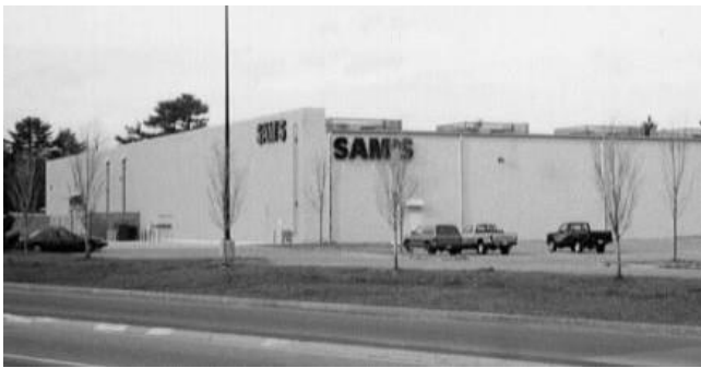
Painted concrete block
