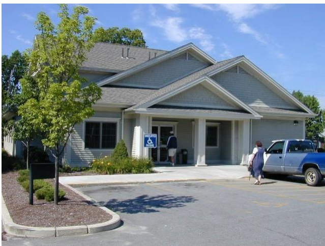
Three views of a branch bank set in a mixed-residential neighborhood. All facades were treated with equal importance. The front (top photo) faces the street and is built to the sidewalk, providing a welcoming presence to pedestrian traffic. The side of the building (middle photo), facing a single family home, is residential in scale and design. The canopy over the rear entrance (bottom photo) provides a transition area between the parking lot and the doorway.
