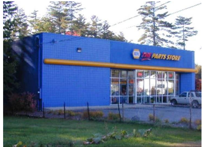
Highly reflective surfaces and bright colors are not characteristic of traditional New England architecture.
