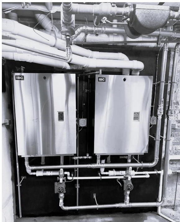
New twin propane boilers at the Leavitt Institute
